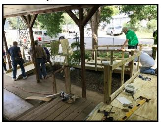
A crew of five to eight people can assemble and install a ramp in about five hours, or one man-hour per foot of finished ramp. Canfield does a lot of the work ahead of time, such as cutting materials and building modules they can carry to the site to assemble.
